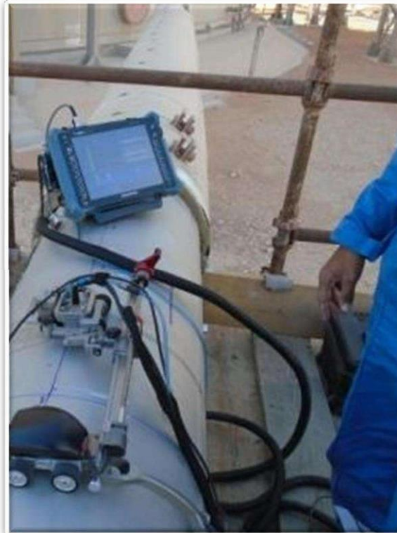
Hydroform Corrosion Mapping - Velosi Oman
