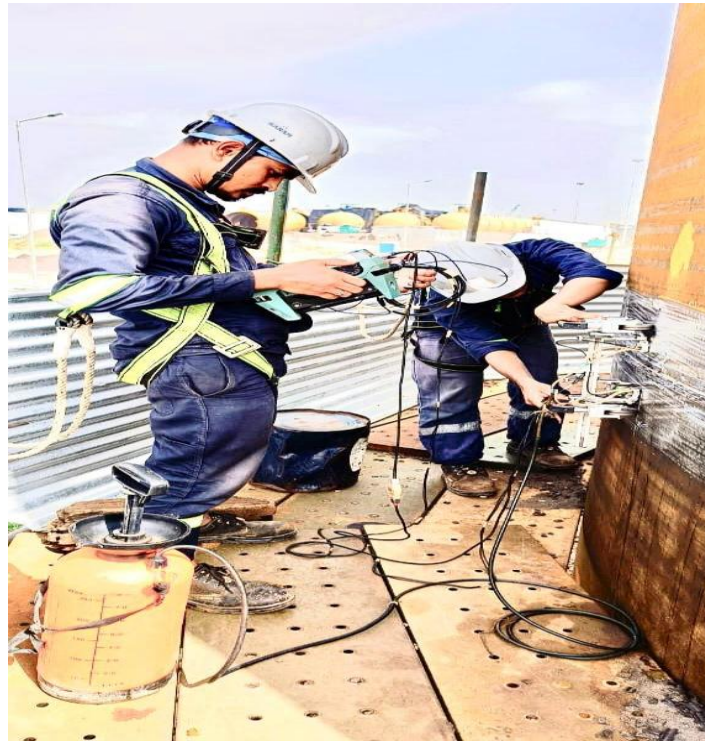
PAUT/ToF Inspection of Mounted Bullets at Vijay Tanks & Vessels, HRRL, Rajasthan, India
