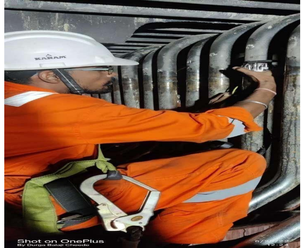
Boiler Tube Inspection at NTPC Ramagundam, Telangana, India
