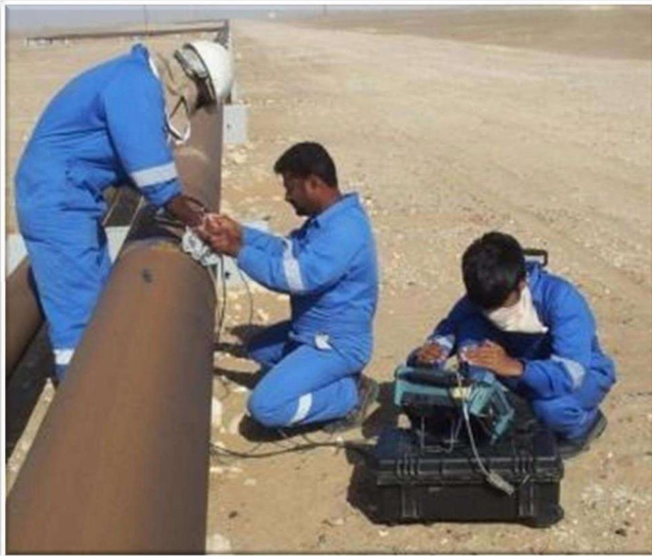
PAUT Inspection Of Pipelines for PDO Oman
